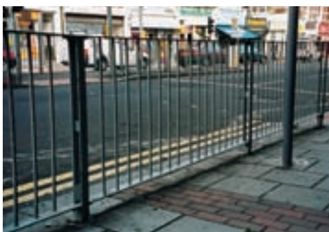
Sometimes facilities introduced in the name of 'pedestrian improvements' actually impede movement on foot and reinforce vehicular priority
