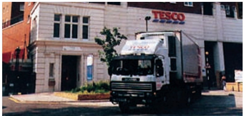
Disturbance caused by reversing lorries should be avoided in designs (here in the otherwise impressive Brook Green flats-over-superstore development in Hammersmith, London)
