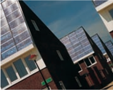
Urban design in the Nieuwland neighbourhood of Amersfoort, Holland, is centred on optimising solar potential
