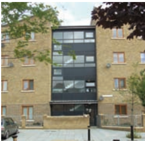
1960s tower blocks have been replaced with a mix of low rise flats and housing
